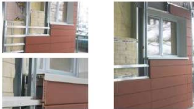
Example of large sized prefabricated steel frame retrofit modu
