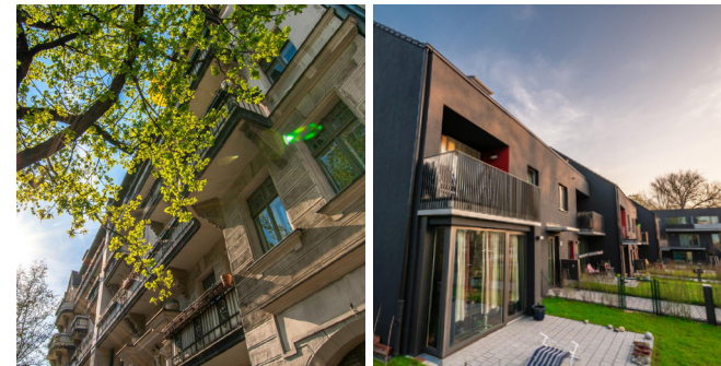
Our very first building in Sickingenstrasse and our current new build in Gartenstadt Falkenberg.
