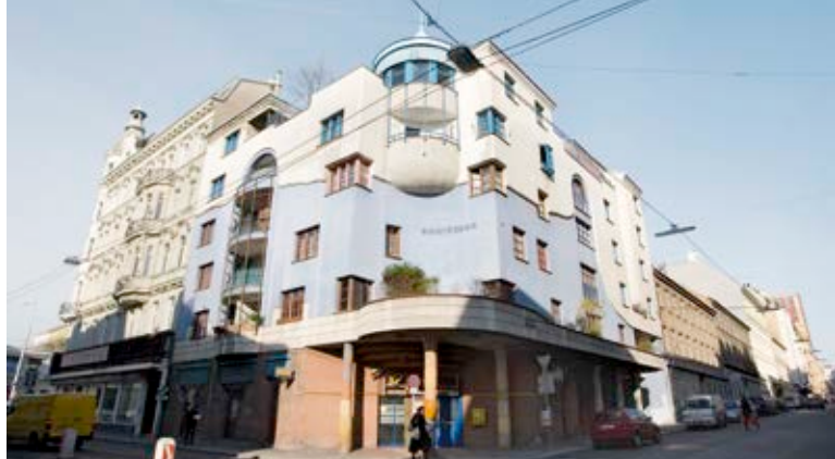
Complex at Wallgasse no. 13, 6 th district
